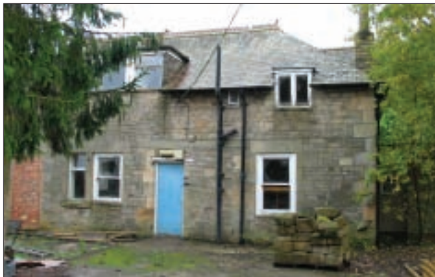
The development site in Allendale
