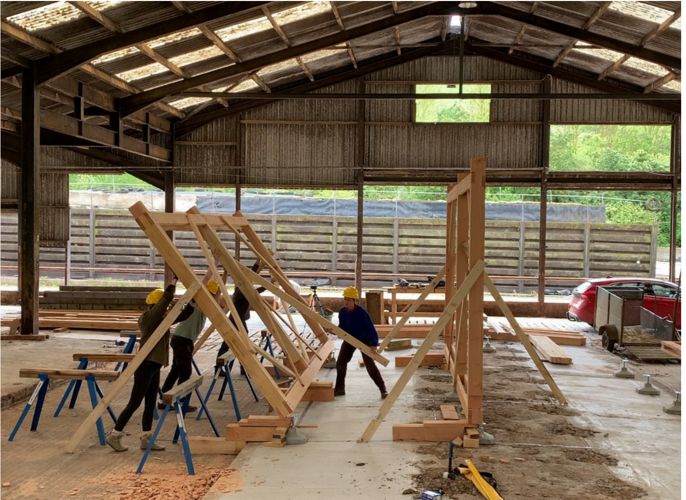
Frames are moved near to foundations on sawhorses and tilted up by four people using props for leverage.
