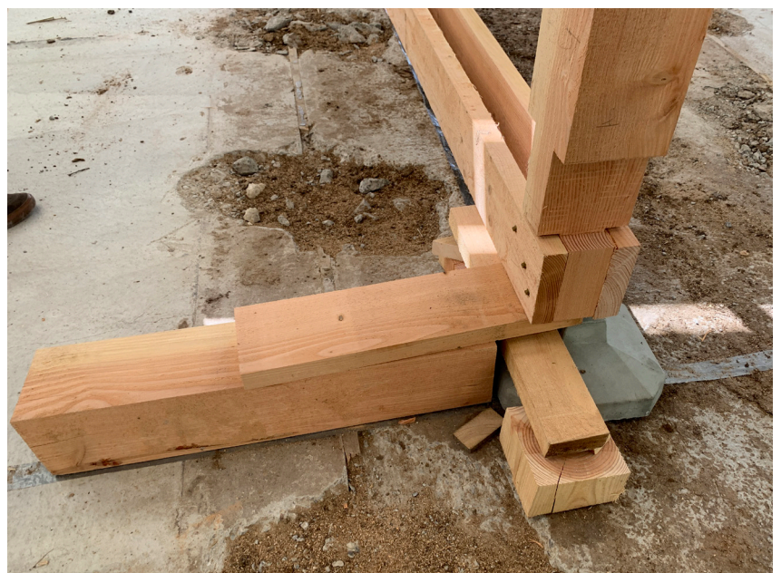
Blocks are shimmed to foundation level to assist with the tilt up.
