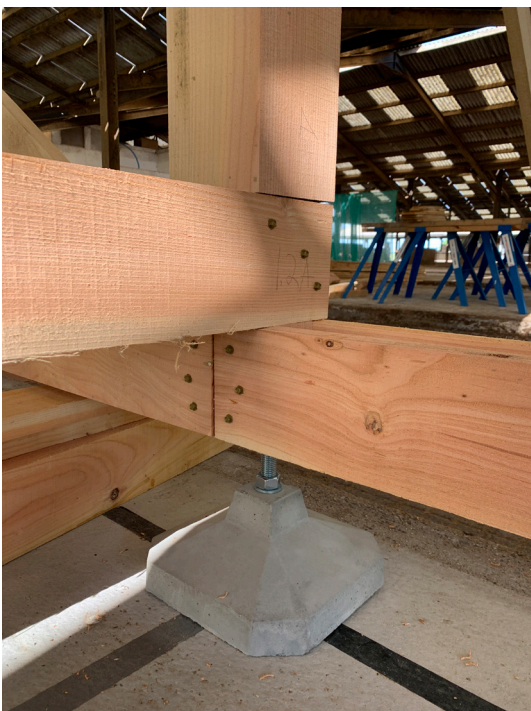
Blocks are shimmed to foundation level to assist with the tilt up.
