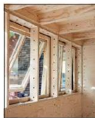
Framed with Cassette Infill Panels
