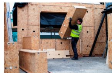
Structural Timber Cassettes
